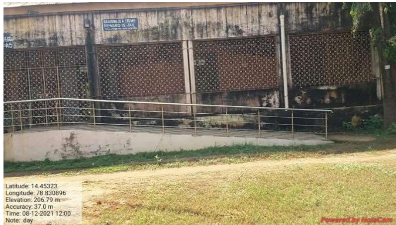
Ramp facility at Auditorium Entrance
